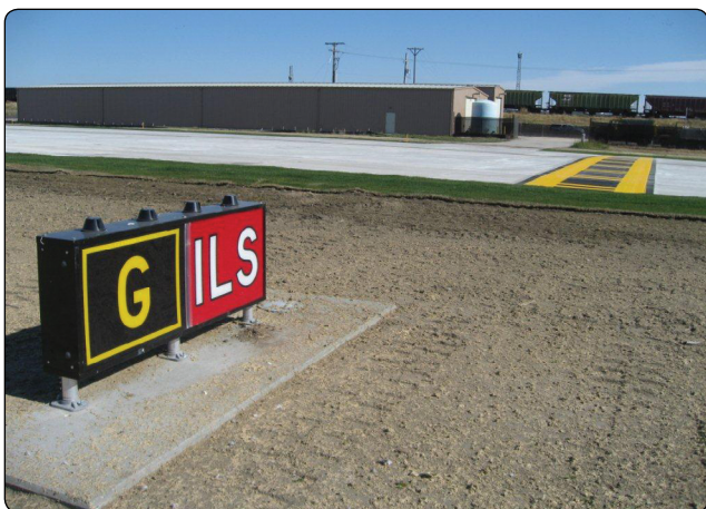
Figure 14-24. Instrument landing system (ILS) holding position sign and marking on Taxiway Golf.
