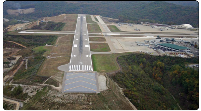
Figure 14-55. Engineered material arresting system (EMAS) located at Yeager Airport, Charleston, West Virginia.
